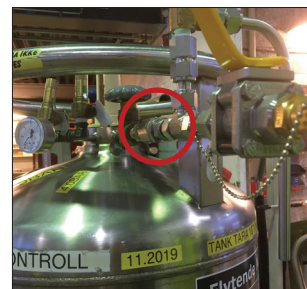
Pressure relief device connected to valve 4
